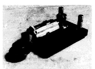
Above is a photo of a key that Rob W2IE made. Specs: all ball bearing, can be adjusted to .0001 inches while in use and reset to a previous setting. Arm weighs 23 grams. Made of 660 bronze, t6 alu, red brass and tiger maple. Rob used to run a design and prototyping firm but now he just plays around, hi. Nice job, Rob!
