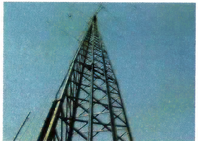
Rotator and beam assembly winched up on “railway lines”!
